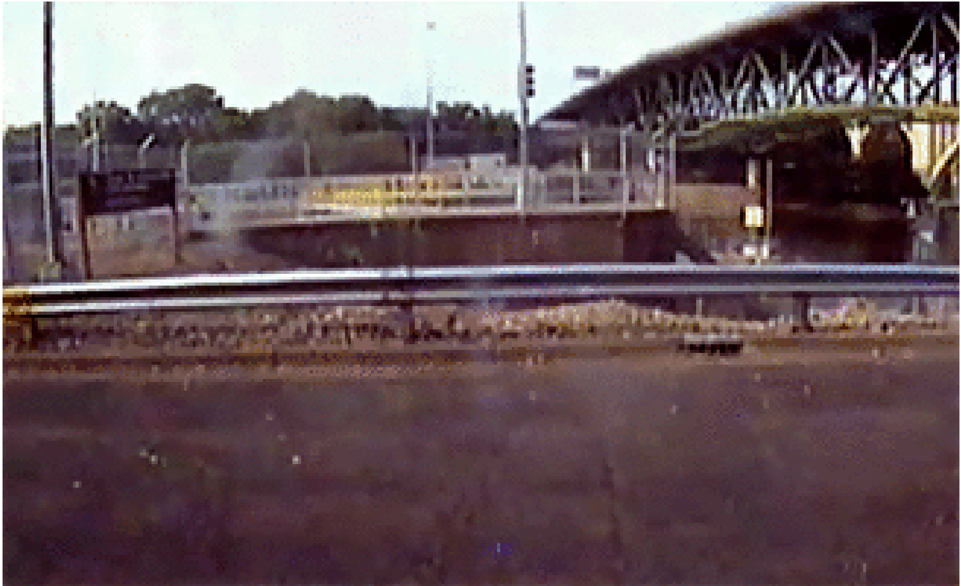
The I35SW bridge collapse on August 1, 2007 at 6:05pm
