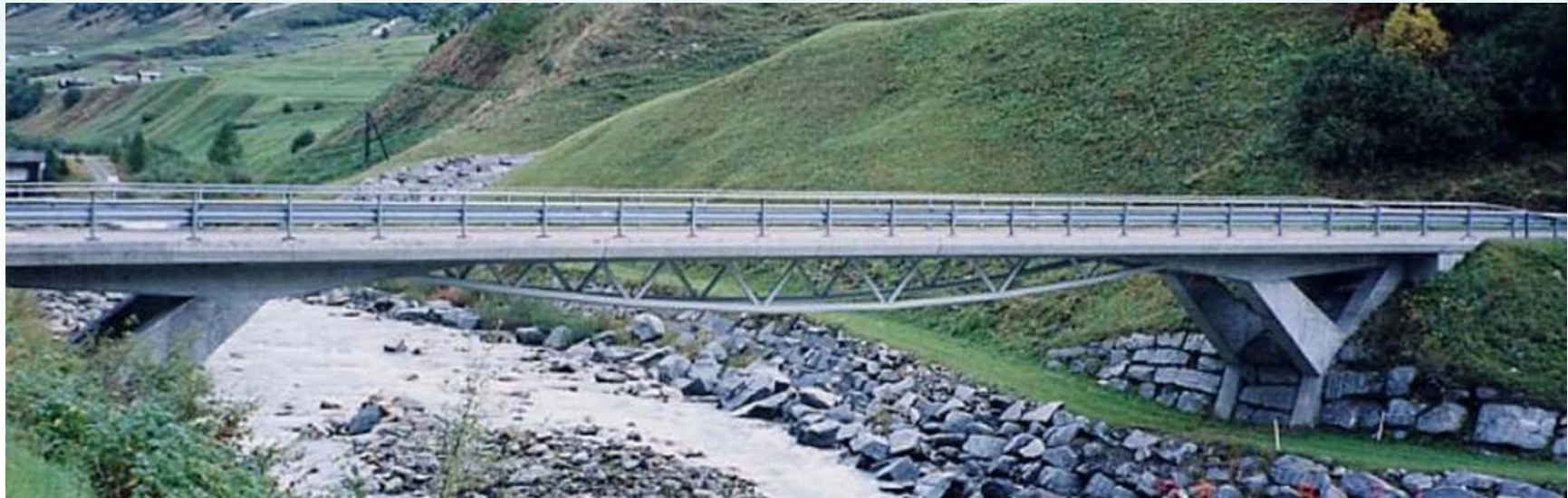
Bedretto Bridge (Ticino, Switzerland)
